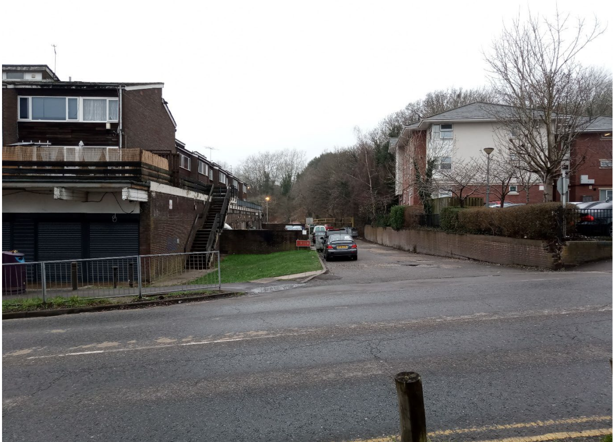
Site visit photograph - existing access at northern site boundary - Victory Close flats to right of image.
